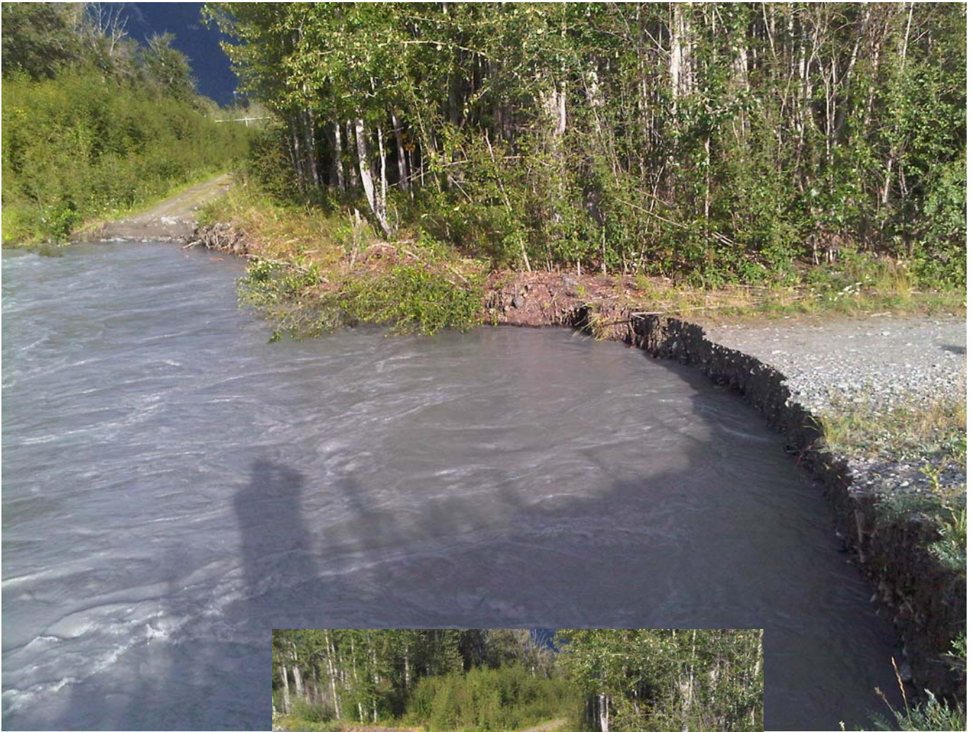
Maud / dike intersection erosion from what was a parking lot and connecting service road to the right.
